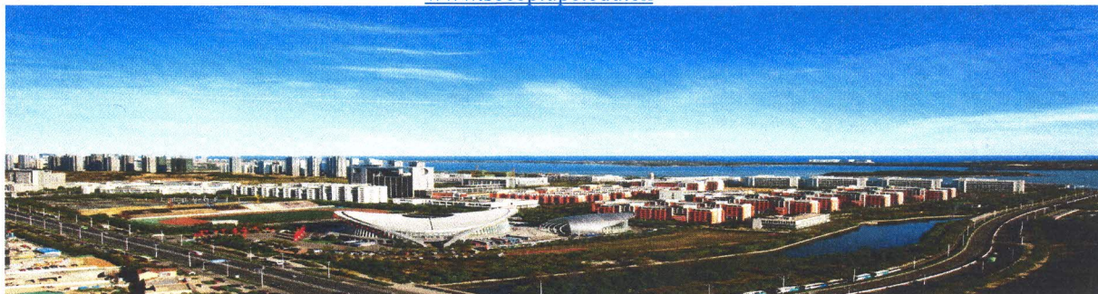
Seashore Campus of China University of Petroleum (East China) in Qingdao
